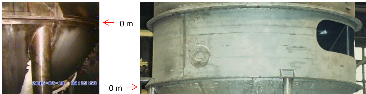
Fig.3. Figure on the left shows visible salt deposits, emanating from where the legs penetrate the vessel insulation. Salt deposits are not visible on or above the support ring (0 m level). Figure on right shows the leg support ring during fabrication before installing vessel interior components, shipping to the site, and installing insulation.
